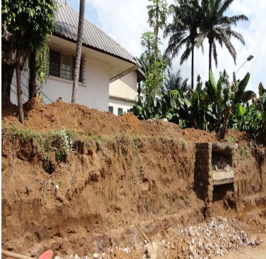
The wall fence collapsed due to Heavy rain.
